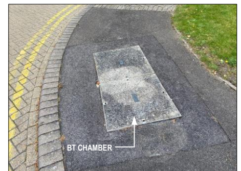
PHOTOGRAPH 3 EXISTING BT CHAMBER IN FOOTWAY ON EAST SIDE OF ACCESS ROAD AT ENTRANCE TO BUILDING CAR PARK
