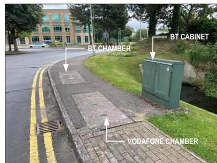
PHOTOGRAPH 2 EXISTING BT CABINET AND CHAMBER PLUS VODAFONE CHAMBER TO WEST OF BUILDING
