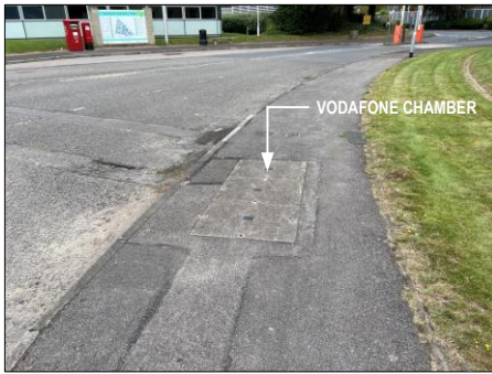
PHOTOGRAPH 4 EXISTING VODAFONE CHAMBER IN FOOTWAY ON EAST SIDE OF ACCESS ROAD TO SOUTH OF BUILDING
